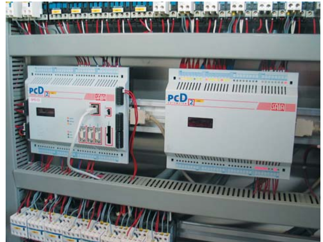
Programmable logic controller PLC of the PCD2 series with MP interface from SAIA-Burgess: building automation with the latest technology
